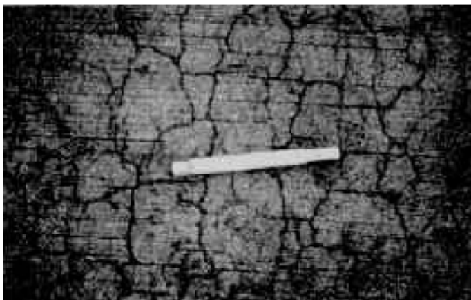
Figure B-10a. Low-Severity Crazing
