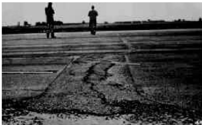
Figure A-16. High-Severity Swell
