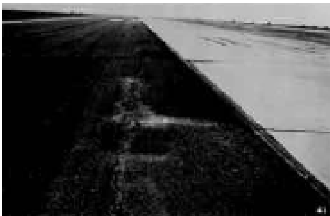
Figure A-14a. Low-Severity Shoving on the Outside and Medium-Severity Shoving in the Middle
