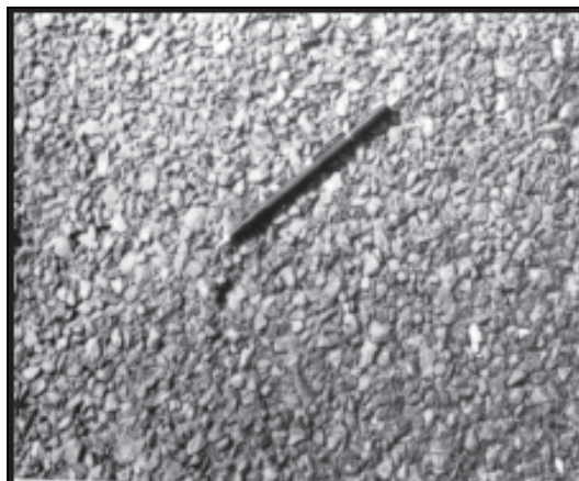
Figure A-12g. Porous Friction Course Low-Severity Raveling and Weathering
