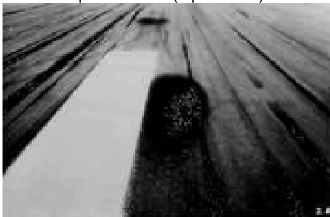
Figure A-6a. Jet Blast Erosion
