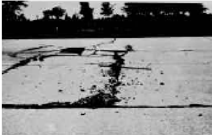
Figure B-1a. Low-Severity Blowup
