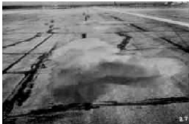
Figure A-5c. High Severity Depression
